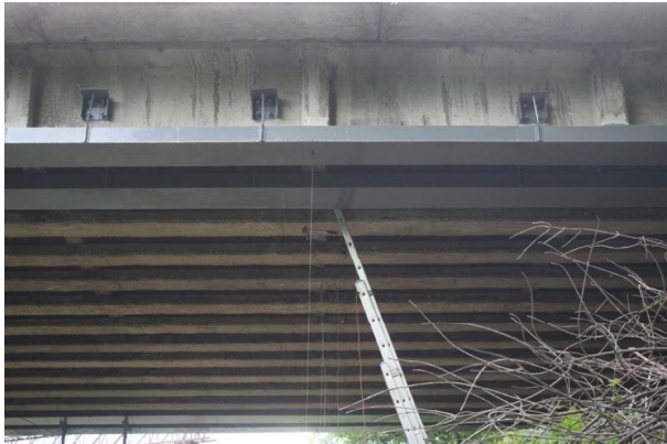
Fig. 3. View of strengthened beams B-13 and B-14, span 3-4
