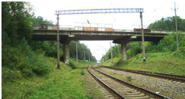
Fig. 1. Left facade of the tested bridge
